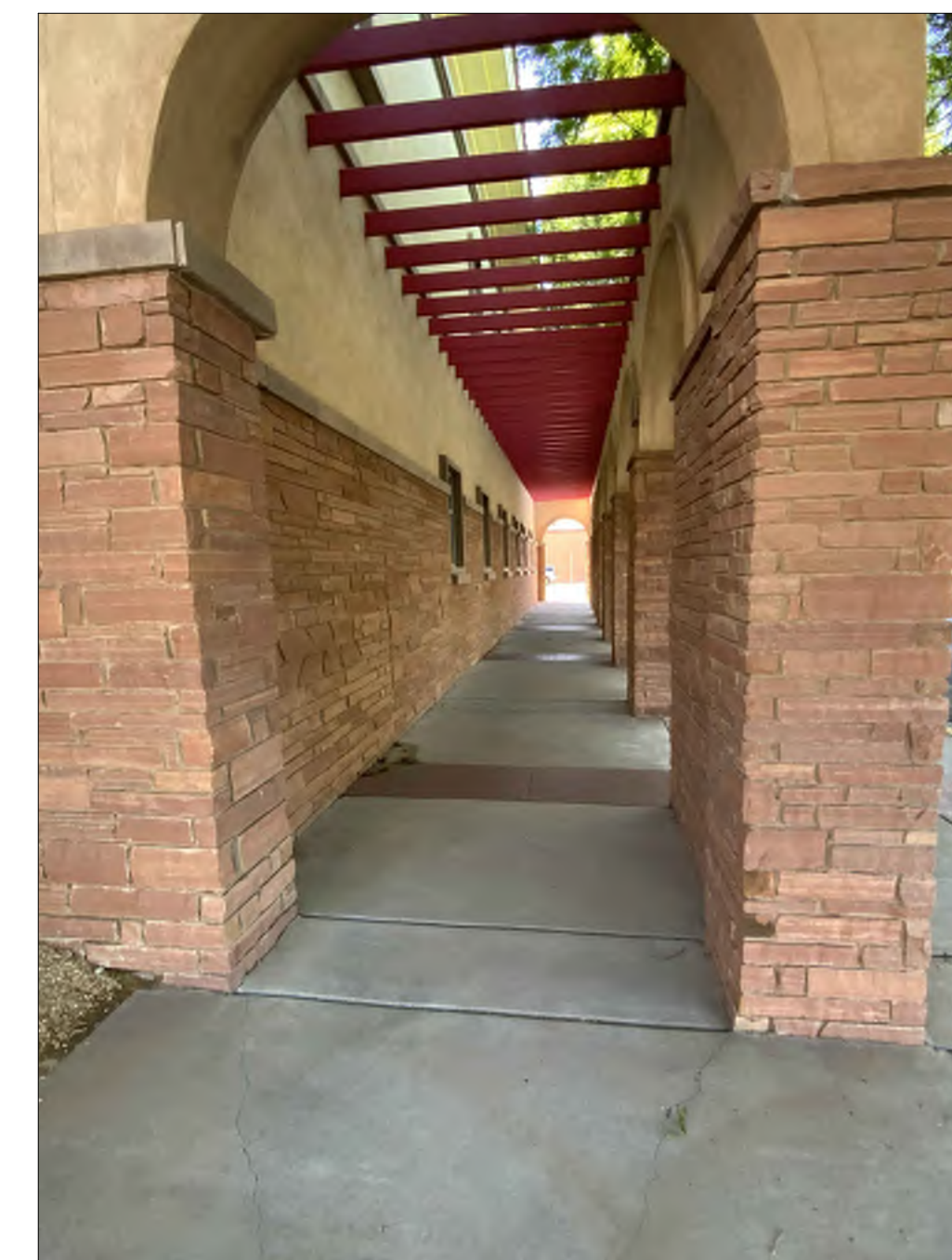
W-4 LOOKING SOUTH
