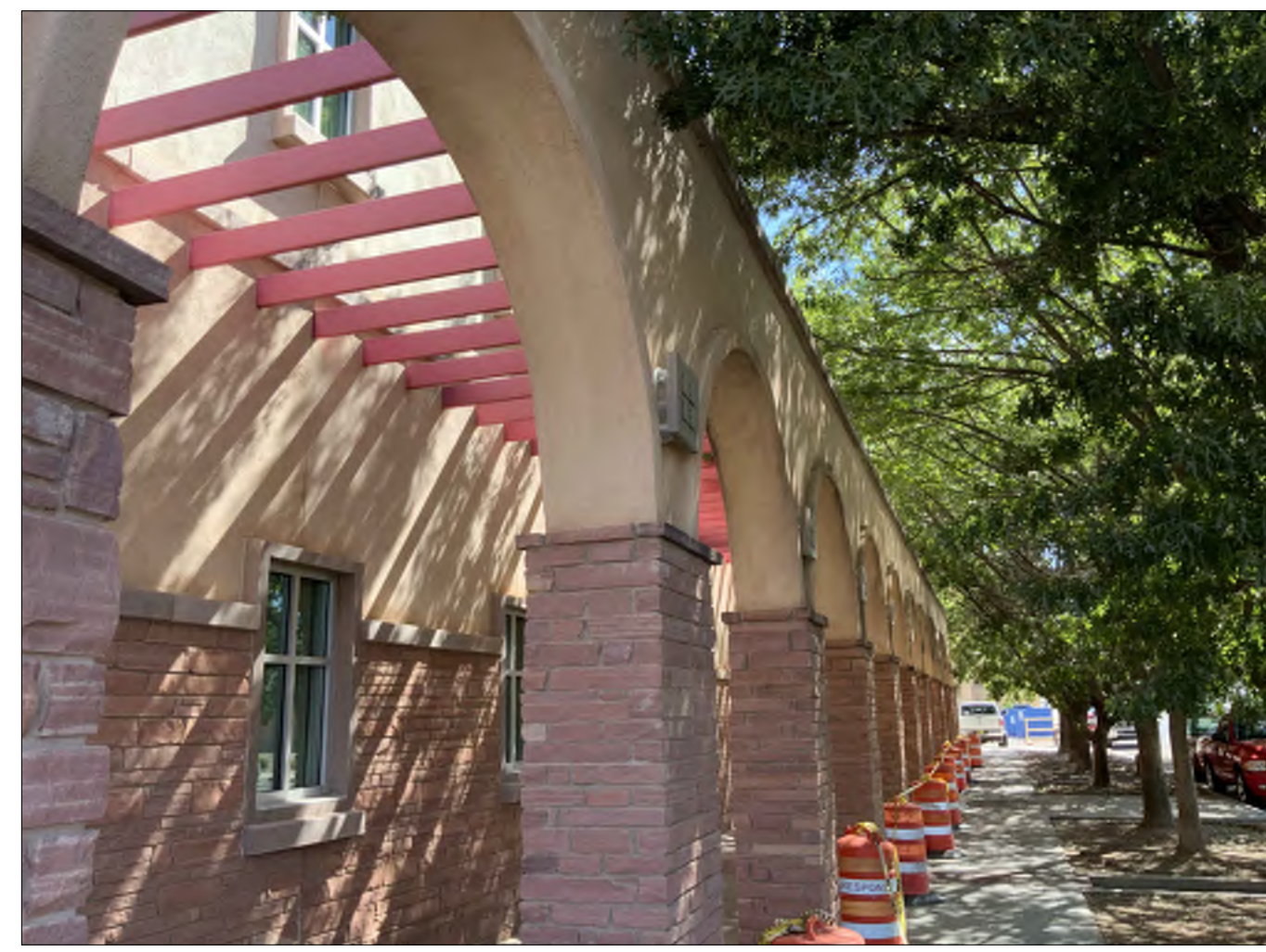
S-1 LOOKING EAST
