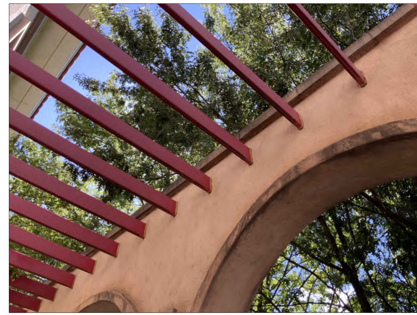
S-3 LOOKING AT TRELLIS BAR SEPARATION
