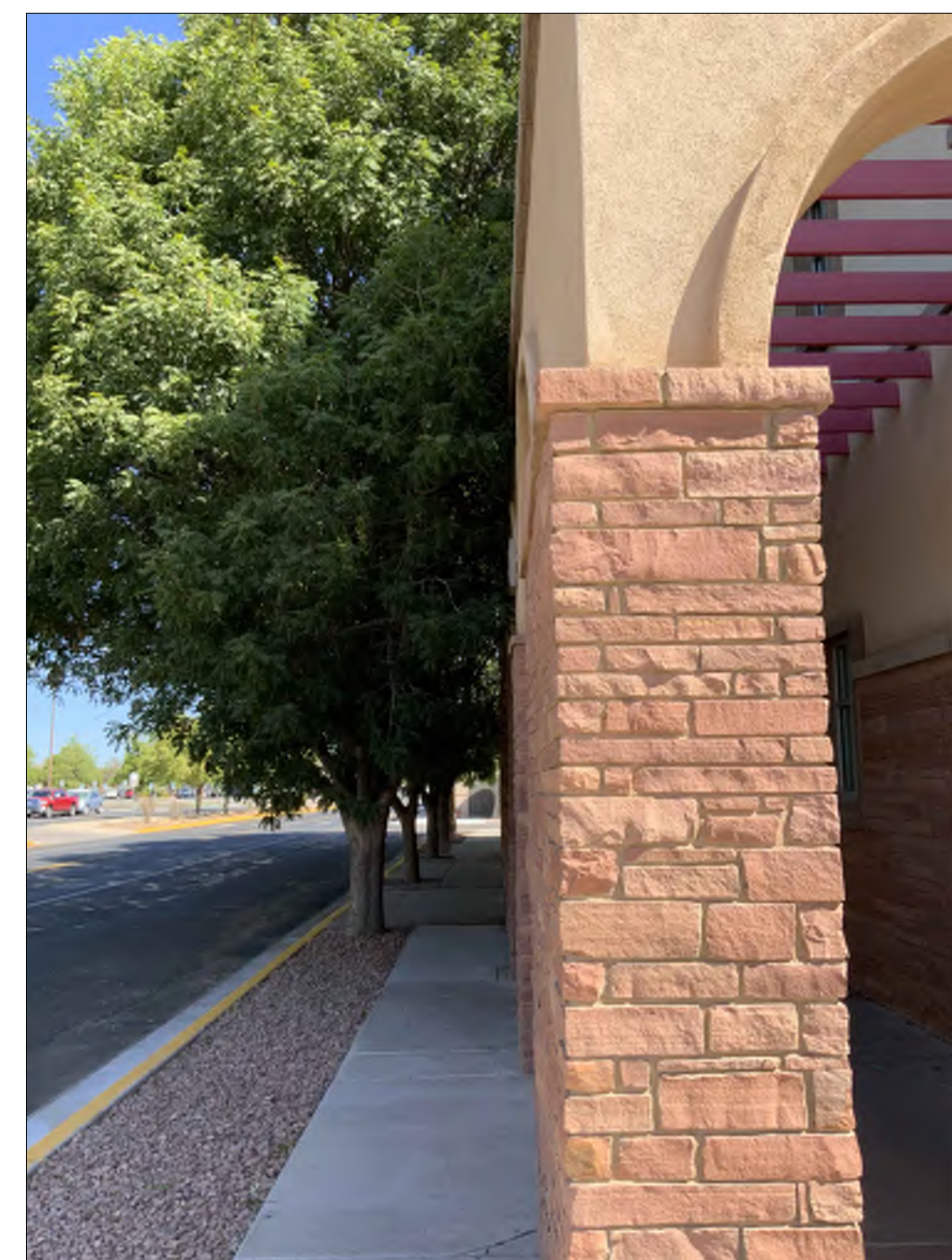
W-1 LOOKING NORTH
